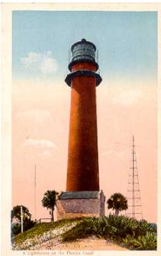
This postcard of the Jupiter Lighthouse shows in good detail the Jupiter Wireless Telegraph Station antenna masts. The mast to the left of the lighthouse was the main and original mast structure and was connected to the lattice tower seen to the right of the light house.
