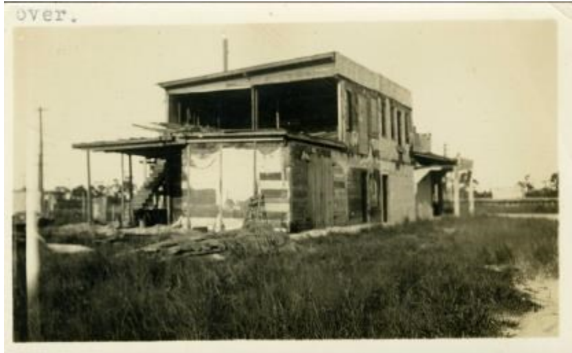
over. Harry Hull Home, Jupiter Florida - Sept 3, 1933 — Hurricane did this — Blew the ends out of 2 bedrooms as shown, part of furniture in field; there was a 2-story porch on front which is gone; blew out all doors and windows, there was another apartment on the end from Martha's and garage underneath.
